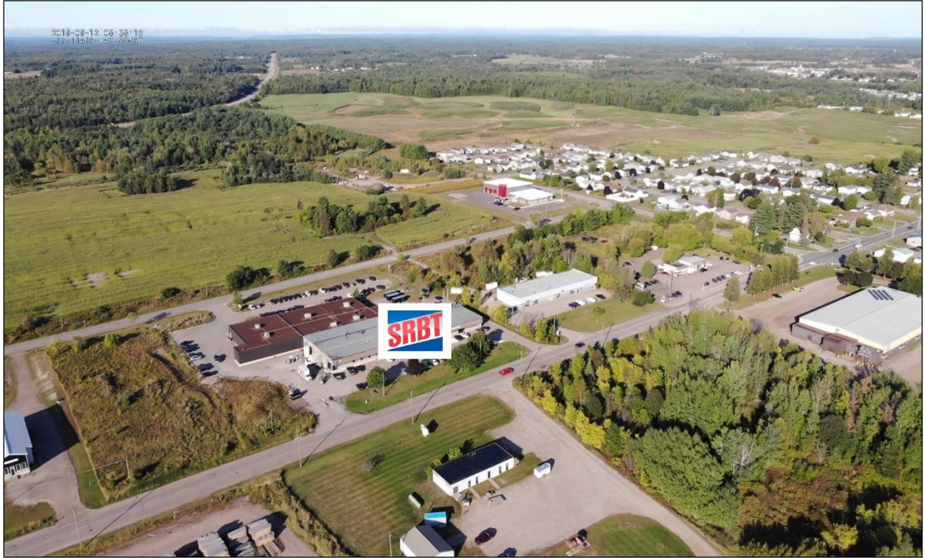
Figure 6: AERIAL PHOTOGRAPH LOOKING NORTHWEST OF SRBT FACILITY
