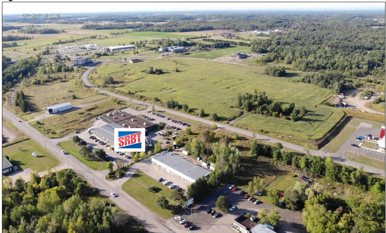
Figure 5: AERIAL PHOTOGRAPH LOOKING SOUTHWEST OF SRBT FACILITY
